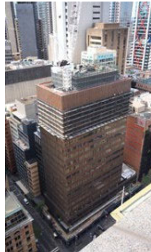
Upgrades begin at 20 Martin Place. Photo: Built
